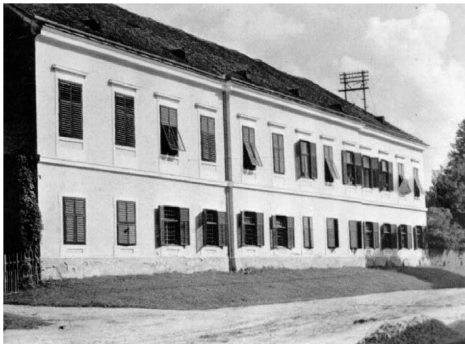
SLIKA 1. Dvorac Kiepach u Križevcima, srušen 1966. nakon urušenja jednog dijela zgrade FIGURE 1. Kiepach Castle in Križevci, demolished in 1966 after the collapse of part of the building
