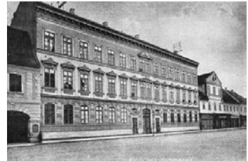
SLIKA 16. Zgrada gimnazije FIGURE 16. High school building
